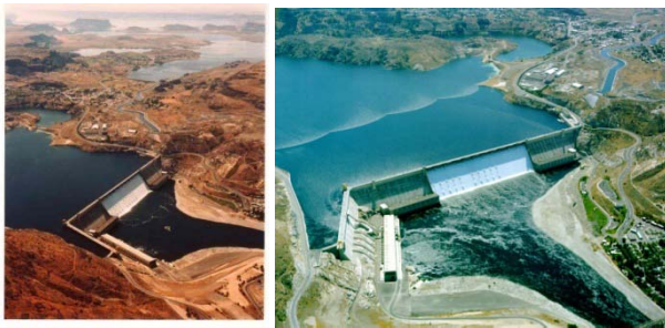
Figure 2 Grand Coulee hydroelectric Plant
